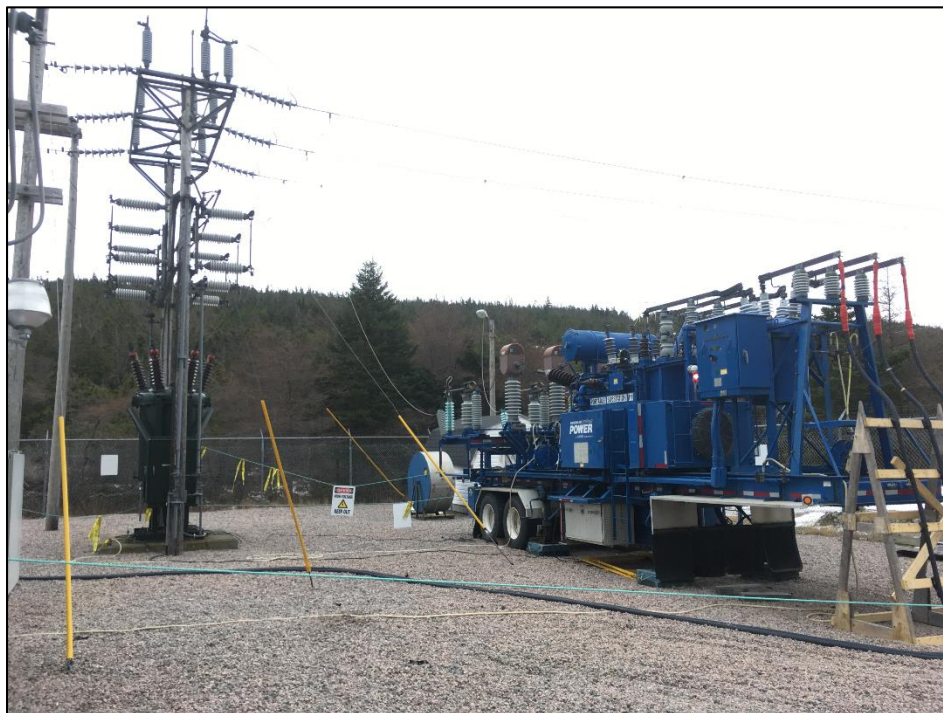
Portable Substation No.1 installed at Riverhead Substation
