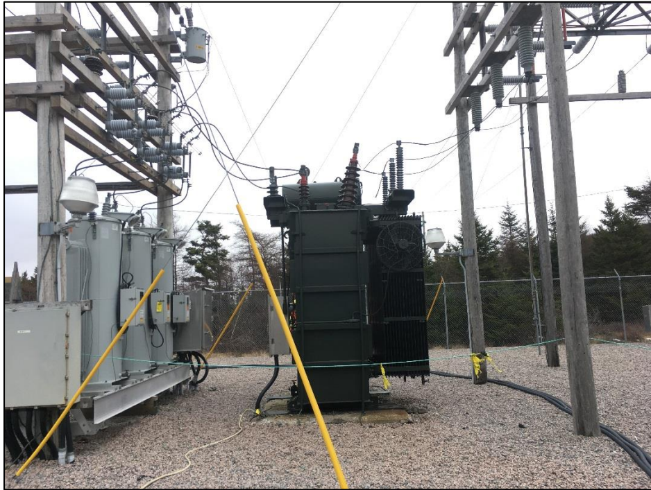
Riverhead Substation RVH-T1 Power Transformer
